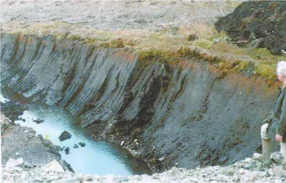
Figure 3: A drainage ditch over 2 metres deep at Cefn Croes wind farm showing surface vegetation, the acrotelm as the light brown upper peat layer about 30cm thick and underneath it the dark brown, waterlogged catotelm
