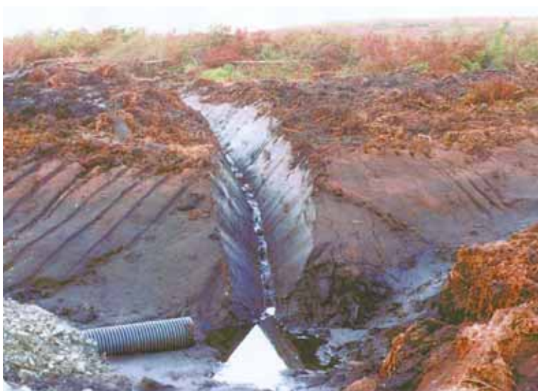
Figure 9: Peat drainage ditches at Cefn Croes wind farm, Wales which will lead ultimately to undercutting, slumping and the breakdown of peat for tens of metres either side of the ditches
